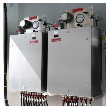
Local electric control cabinets inside the container with EXP-specification according to CSA.
