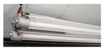
Lighting inside the container including switches, cable and cable glands according to CSA EX-Specifications.
