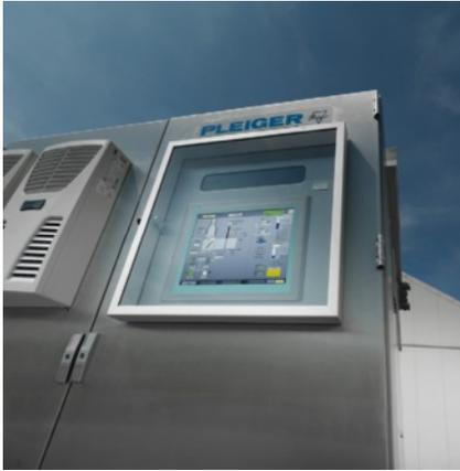
Hydraulic power unit (HPU) with daylight-readable MP377; The hydraulic power units (HPUs) by Pleiger Maschinenbau are responsible for the diverter damper's controlled opening and closing and for its emergency operation, e. g. in case of power failures.
